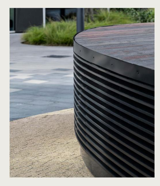
The individual profiles even make it possible to use Linarte to finish curved façades with a minimum radius of 800 mm.
